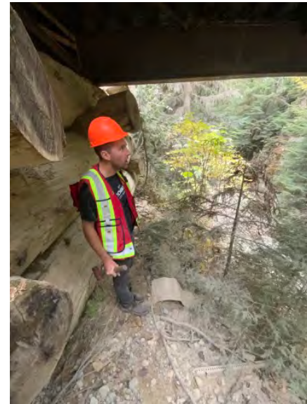
Left Bank Abutment when facing downstream
