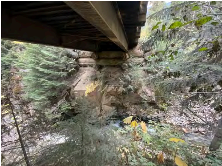
Right Bank Abutment when facing downstream
